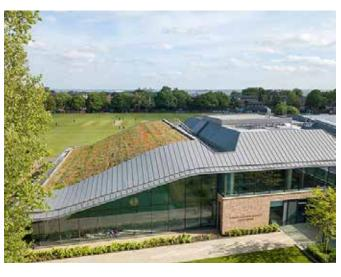
Metal Cladding: A choice of cladding materials to blend harmoniously with the natural timber cladding and break up the building mass.
